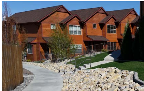
Figure 3.10 Exterior finish building materials should be of a nature in color and texture that is complimentary with the structures within each building district.
